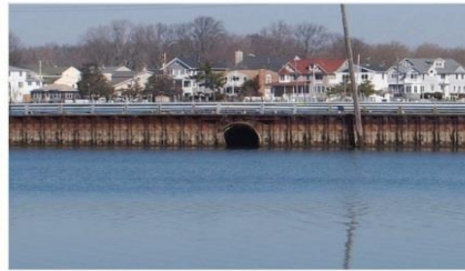
Fisk Avenue Culvert (W-8) between Debbie's Creek and The Glimmer Glass
