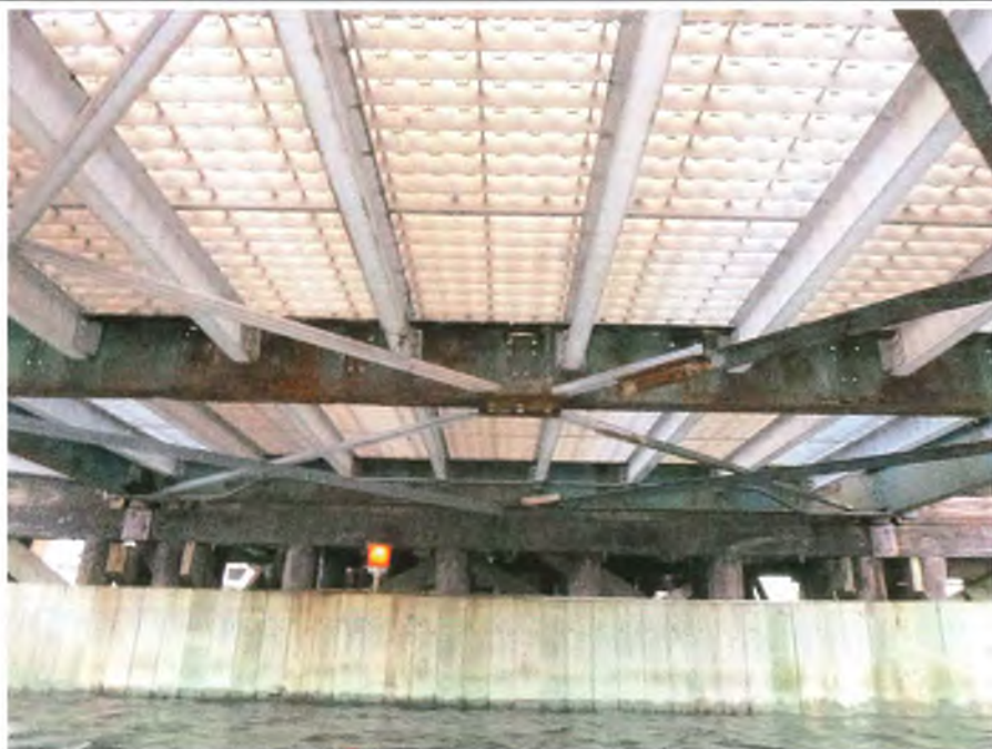
Photo 7 Category: 00 - General View Description: Span 6 (lift span), looking west.
