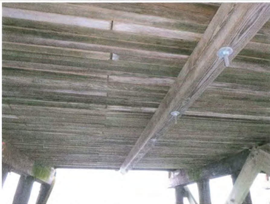
Photo 8 Category: 00 - General View Description: Typical approach span superstructure (Span 3), looking south.
