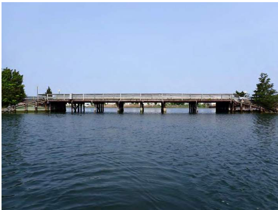
Photo 2 Category: 00 - General View Description: East elevation, looking west.
