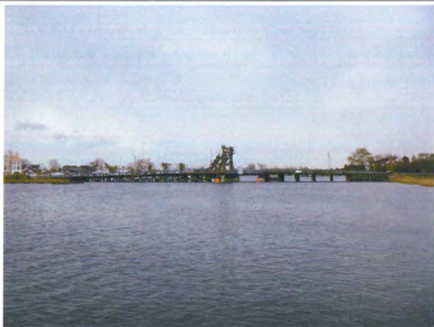
Photo 2 Category: 00 - General View Description: North (flood) elevation, looking south.
