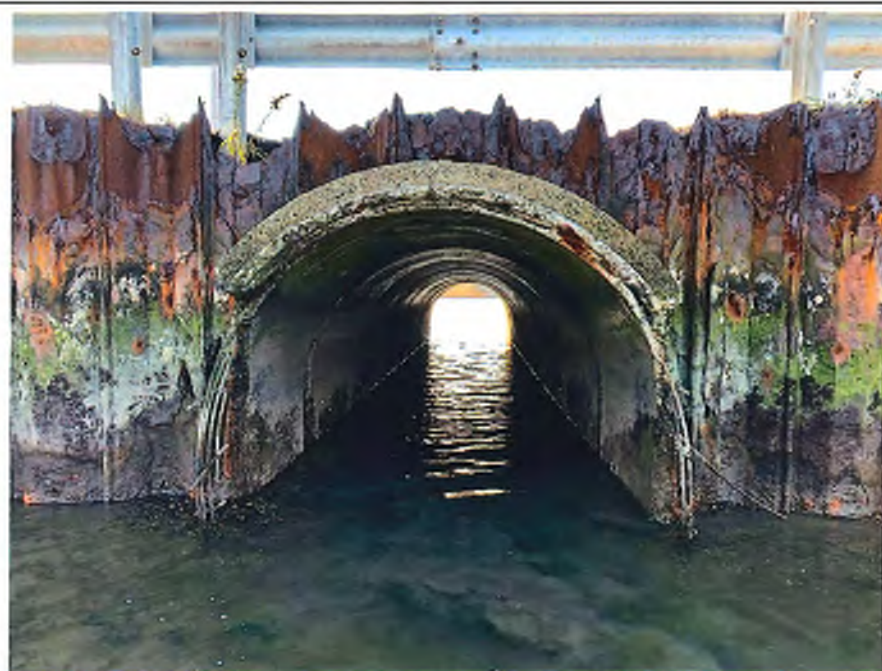
Photo 1 Category: 00 - General View Description: West elevation, looking east.
