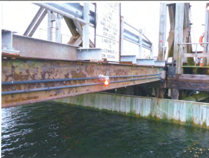
Photo 42 Category: 61 - Work Done, 39 - Fender System/Navigation Lighting
