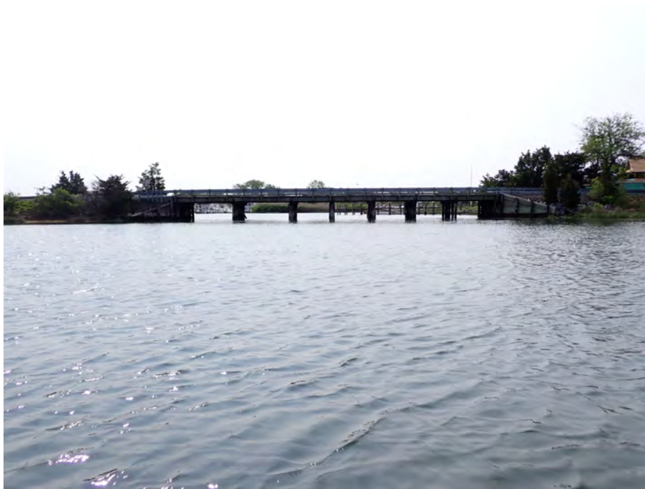
Photo 1 Category: 00 - General View Description: West elevation, looking east.
