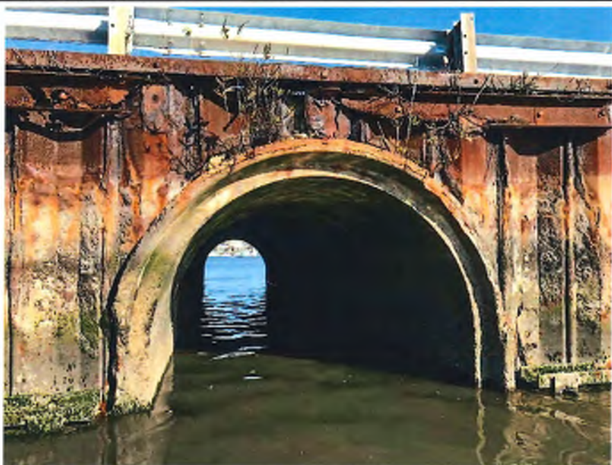
Photo 2 Category: 00 - General View Description: East elevation, looking west.
