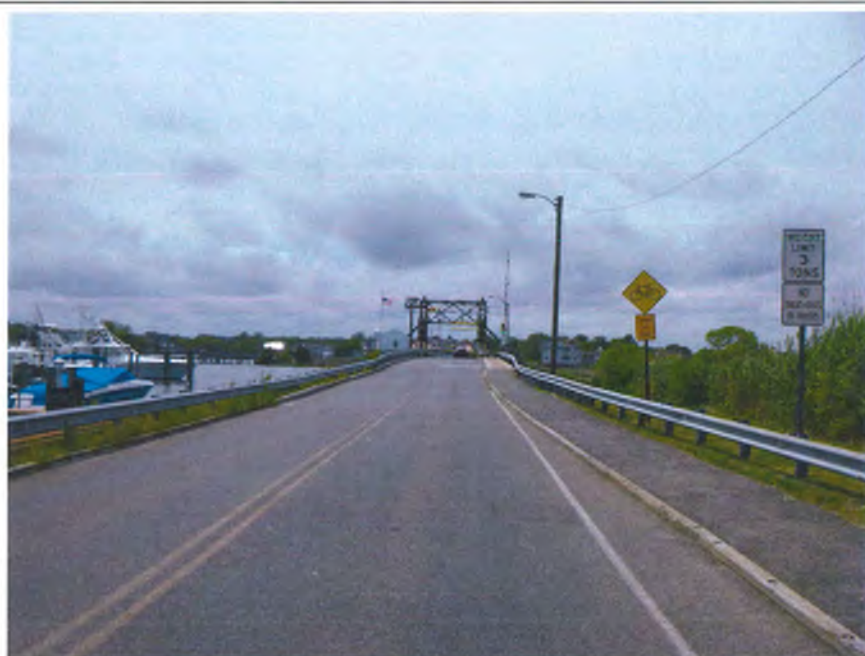
Photo 3 Category: 00 - General View, 02 - Approaches Description: East approach roadway, looking west. There is no barrier gate at the east approach.
