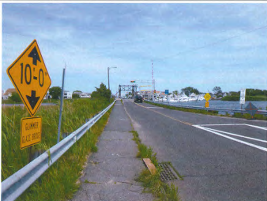
Photo 40 Category: 10 - Signs/Posting Description: West approach, looking east. 3 Ton Weight Limit sign and 10 ft Vertical Clearance sign.
