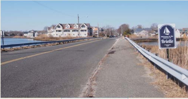
Fisk Avenue, looking west
