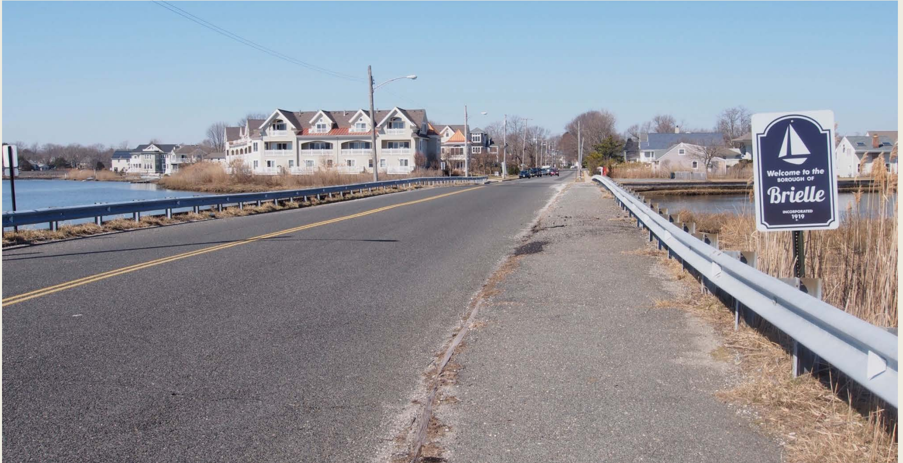
Fisk Avenue, looking west
