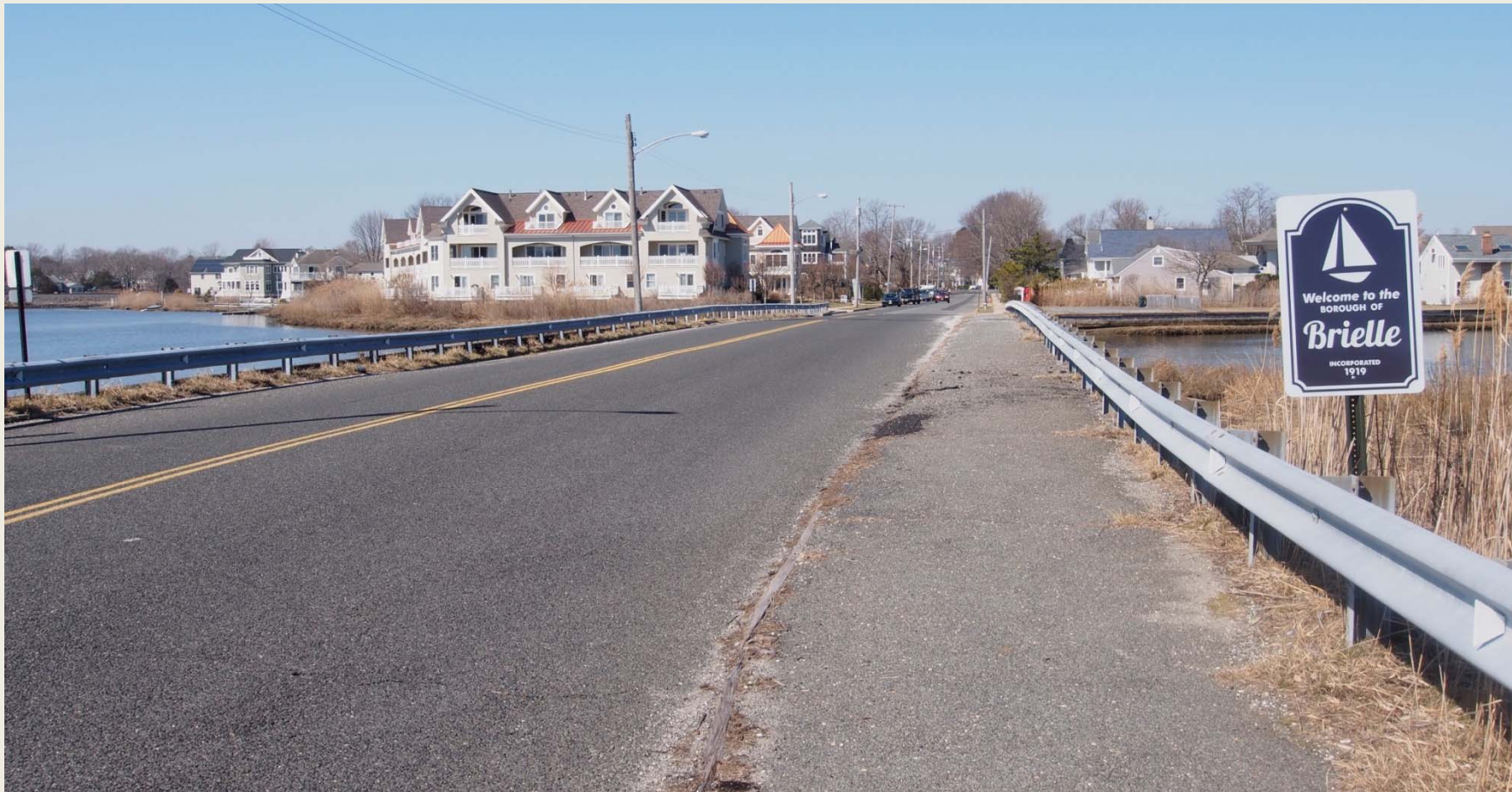
Fisk Avenue, looking west
