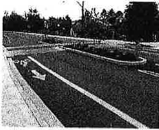
Median island with a raised mid-block pedestrian crossing
