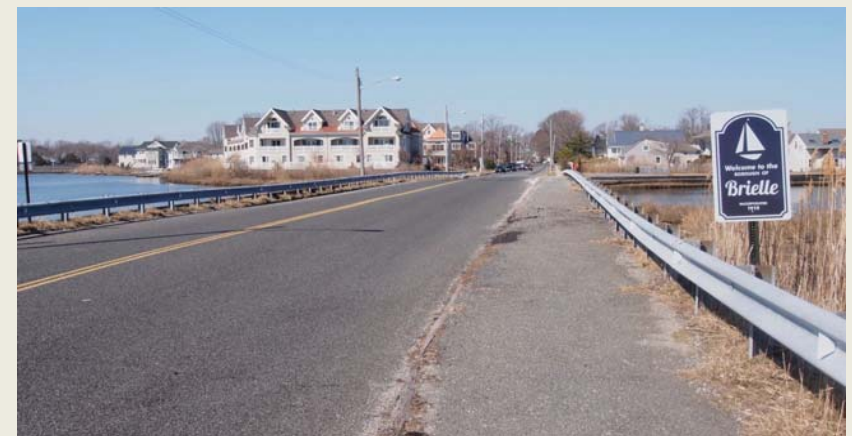
Fisk Avenue, looking west
