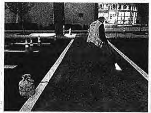
Construction of polymer cement overlay to change asphalt to brick texture and color to indicate high traffic crosswalk
