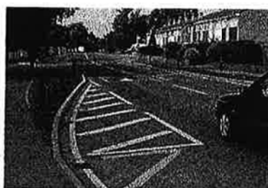
Two traffic calming measures: speed cushions (the two reddish pads in the road) and a curb extension (marked by the black posts and white stripes)
