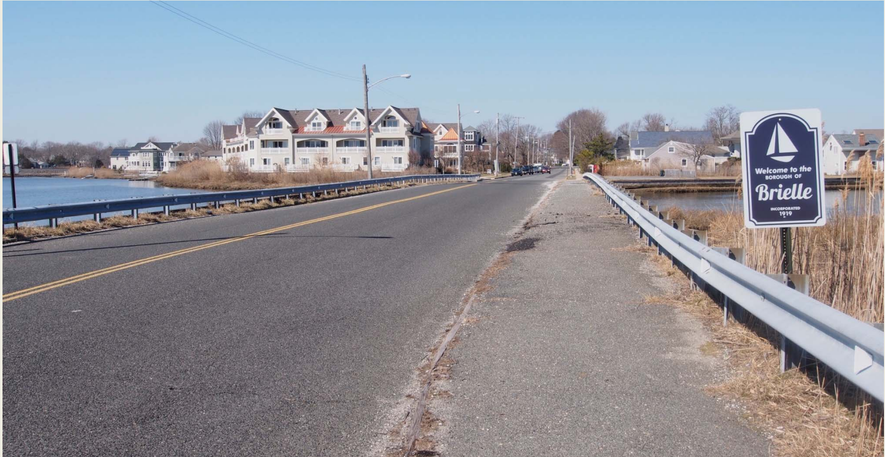
Fisk Avenue, looking west
