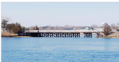
Green Avenue over Debbie's Creek (W-7)
