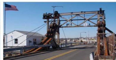
Brielle Road over The Glimmer Glass (W-9)
