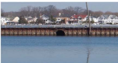
Fisk Avenue Culvert (W-8) between Debbie's Creek and The Glimmer Glass
