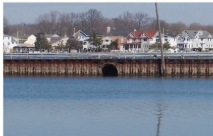
Fisk Avenue Culvert (W-8) between Debbie's Creek and The Glimmer Glass
