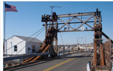
Brielle Road over The Glimmer Glass (W-9)
