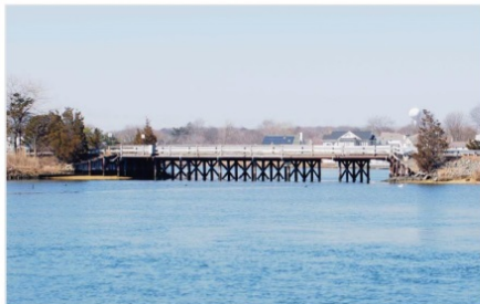
Green Avenue over Debbie's Creek (W-7)
